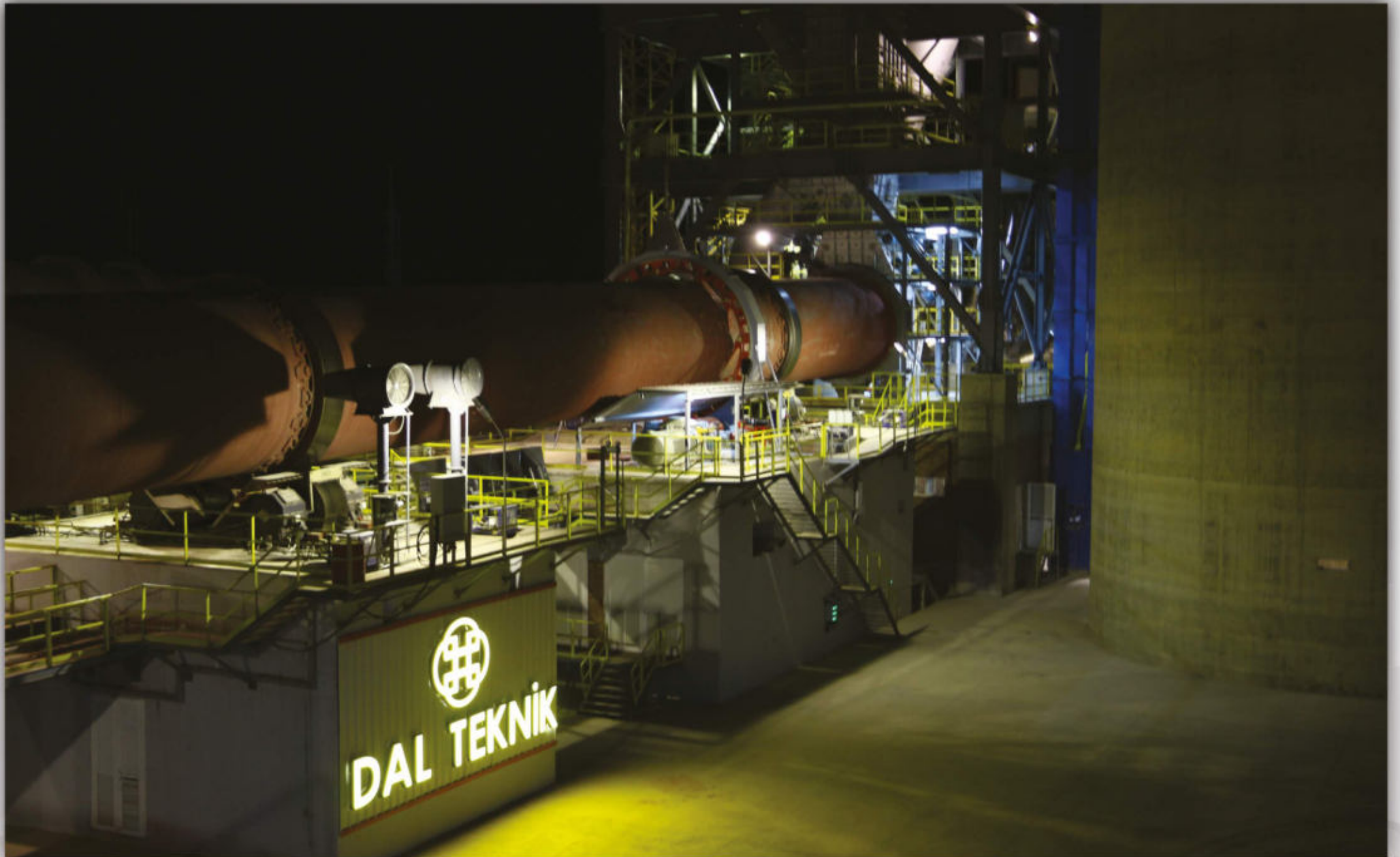
Rotary Kiln - Uzbekistan
